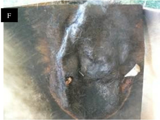
A close up of the rear of the pane, showing the burn through holes and distortion.
